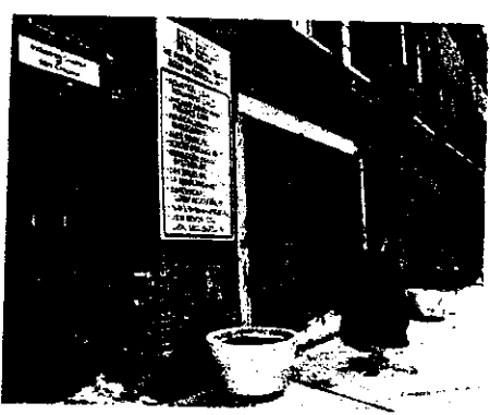
Georgia Tech's Advanced Technology Development Center occupies a new building (right). More typical is the Fulton-Carroll Center for Industry in Chicago, in three old warehouses.
